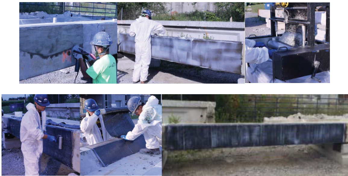
Figure 53 – FRP Application to Damaged PC Girder C
