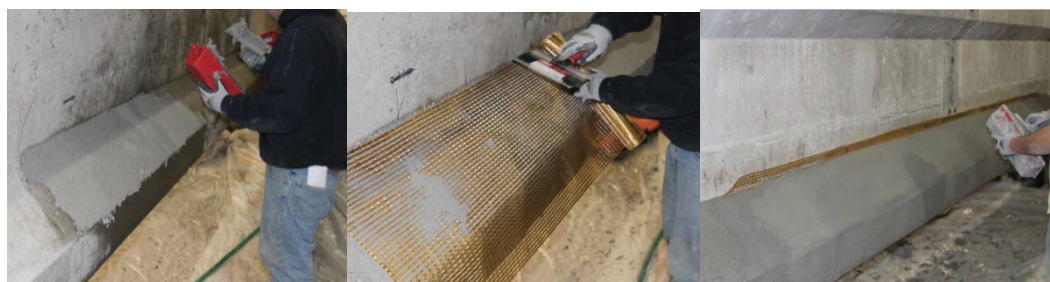
Figure 55 – FRP Application to Damaged PC Girder C
