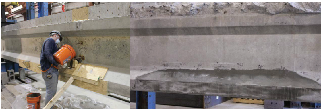
Figure 46 – a) Concrete Repair Formwork b) Repaired Area
